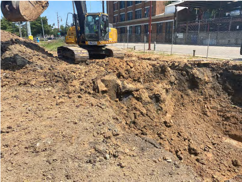
Photo 2: View of a sump encountered during soil removal on the west portion of the Site (facing southeast).
