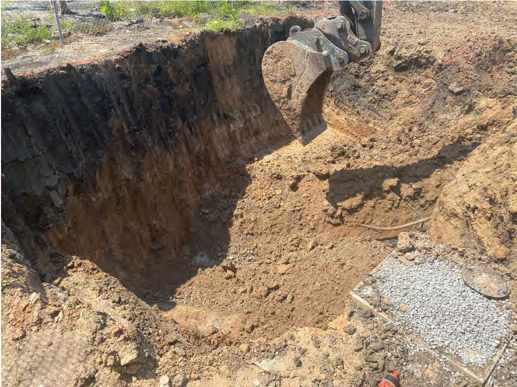
Photo 6: View of excavation near SB-02/MW-02 prior to its removal (facing north).
