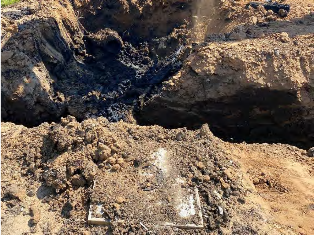
Photo 4: View of a pipe connected to the sump and oily staining north of SB-02/MW-02 (facing northeast).
