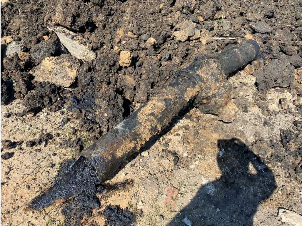
Photo 5: View of the removed pipe (facing southeast).
