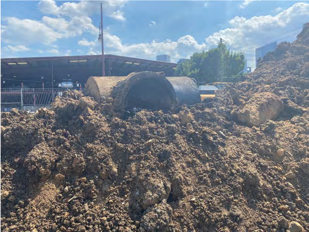
Photo 3: View of the removed sump and soil stockpile (facing southwest).
